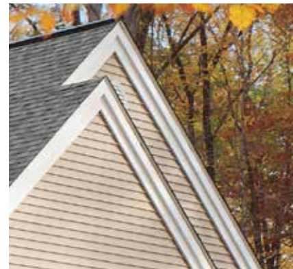
5" Trimworks lineals used as "rake" boards.
