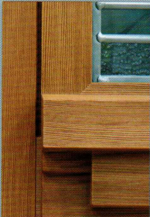
Details of the Craftsman Fir Grain Construction
